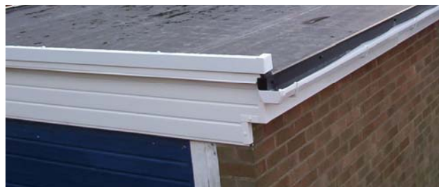
Photograph shows finished Edge & Gutter Trim
