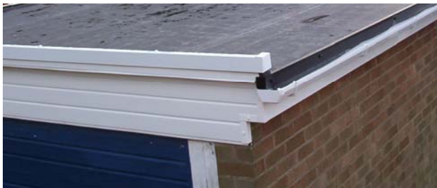
Photograph shows finished Edge & Gutter Trim
